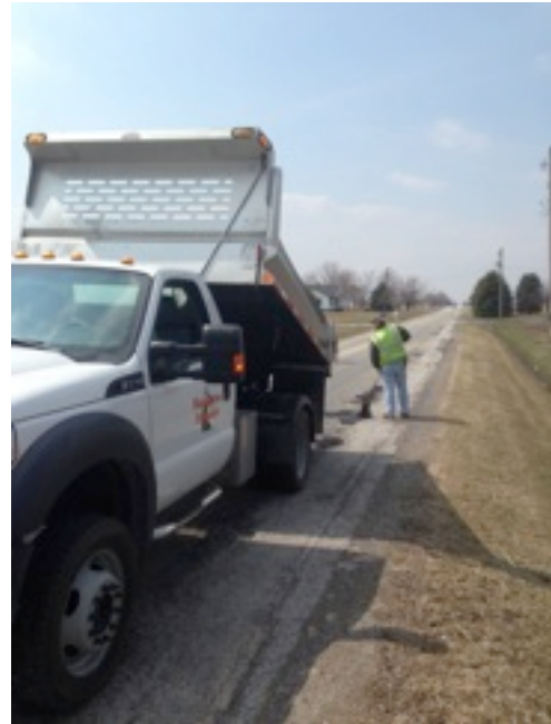
A Road District employee is busy patching small holes on township roads. The severe winter took a huge toll on ALL roads throughout the state.
