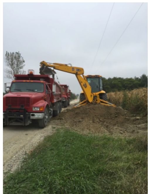
Corning Road Ditch Work
